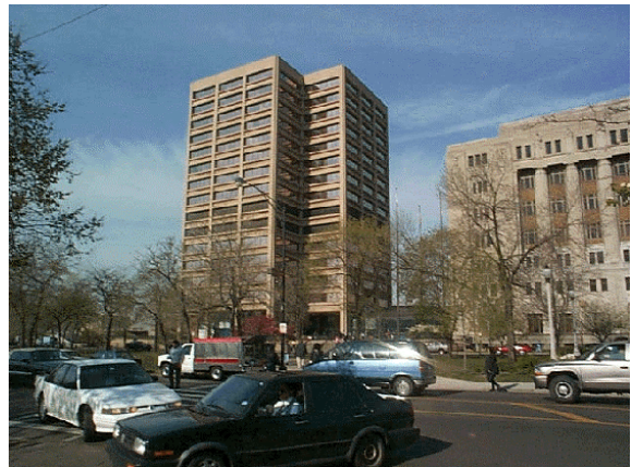
Cook County Criminal Court Administration and Courthouse Buildings
